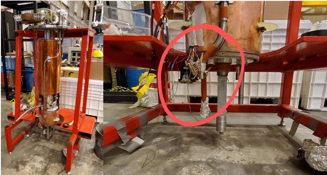
Turret with cover removed (left), connectors to be repaired (right)
